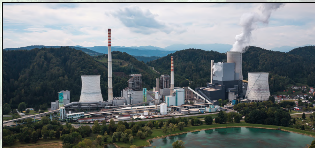
Figure 1: Šoštanj Thermal Power Plant
